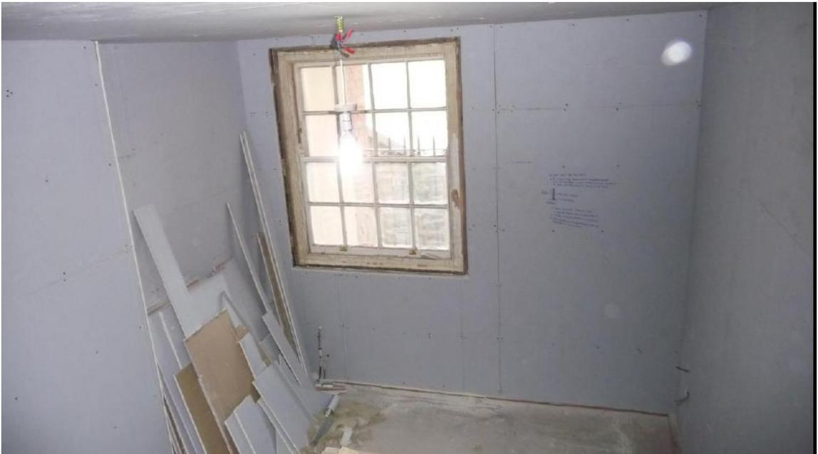
This shows the finished walls and ceiling, apart from around the window. Please note the gap at the very bottom of the plasterboard at floor level. This should be sealed with permanently flexible sealant. The plasterboard joints and screw heads are then sealed as normal. The skirting board should have a very small gap between it and the floor to reduce the risk of flanking sound.
