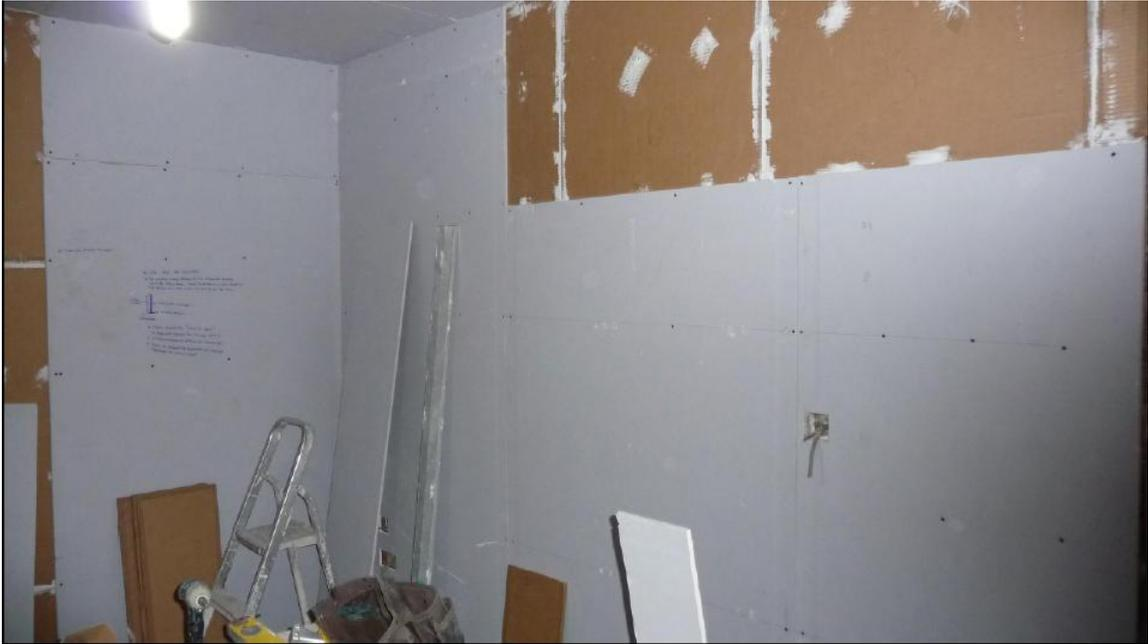
Acoustic plasterboard is then secured by screwing into the resilient bars only, using 38-42mm drywall screws. If possible use a brickwork pattern. If you are only treating the walls and not the ceiling then leave a 5mm gap all around the perimeter edges and seal this gap with permanently flexible sealant. In this case the ceilings and walls have both been upgraded to create an acoustic seal, so the plasterboard can go into the corners.
