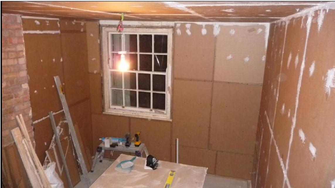
The PhoneStar boards can optionally be sealed with flexible sealant at the joints and perimeter, to ensure there are no gaps to allow sound to escape through. The screw heads are also sealed in this case.
