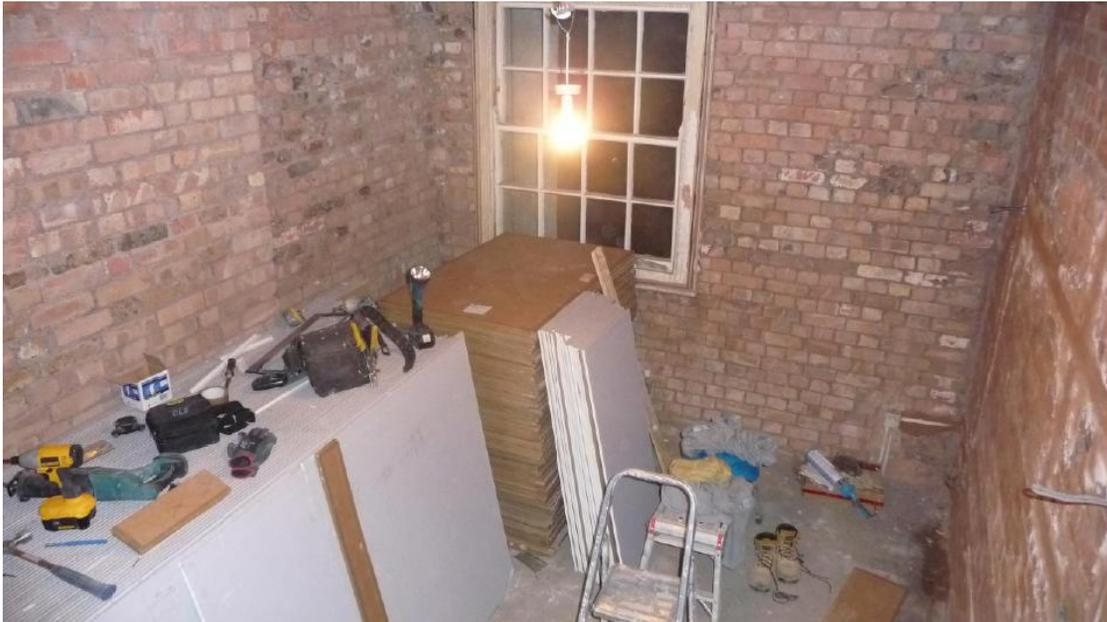
These walls have been stripped back to the bare bricks. Although this is not necessary it allows the installer to seal any gaps in the mortar or around electric wiring as well as all the perimeter edges. In addition it saves living space.
